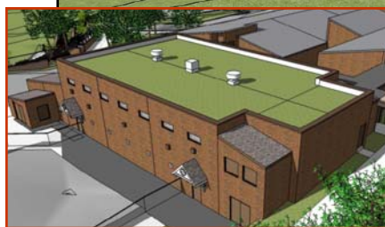
A three-tiered micro-bioretenion area and a green roof are part of the addition of a new gymnasium at Cold Spring Elementary School in Montgomery County.
